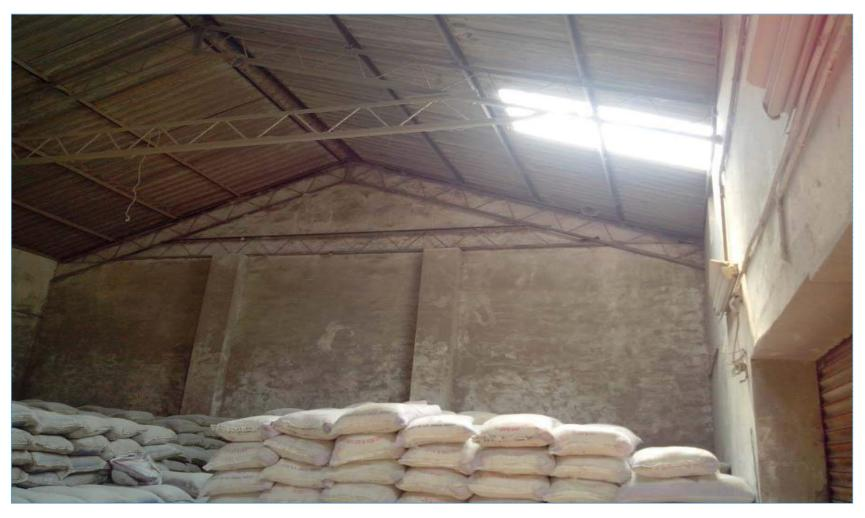
**Increasing Usage of Natural Light by Using Transparent Sheet on Roof**
