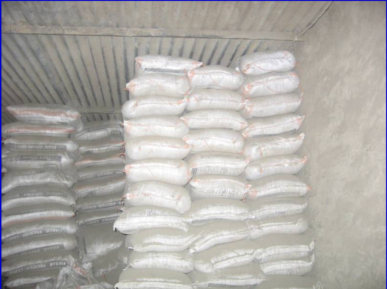
Cement storage – Loading against wall, loading up to the ceiling
