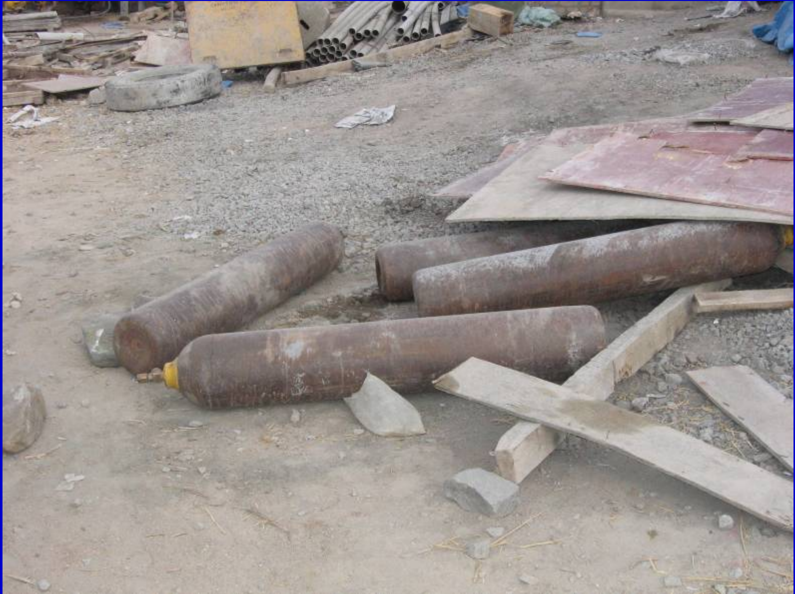
Gas cylinder kept horizontally anywhere
