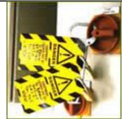
If the electrical power has been turned off to allow you to do work safely, it is essential that the power stays off until you have finished work. Make sure YOU are in control and STAY in control. A good way is to have the only key to the switch or a locked room or cabinet containing the switch. Remember, if you remove a fuse, another one could be inserted in its place, and people ignore notices. If you have any doubts that the electricity may be turned on again without you agreeing, STOP WORK.
