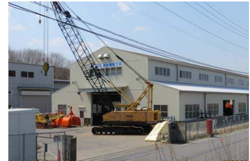
Main entrance of the plant No1
