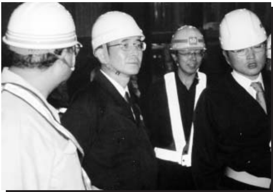
Mr. Hisami OKUDA (second from left), Director, Tokyo Labour Office, personally provides guidance at a construction site (October 4, 2004).
