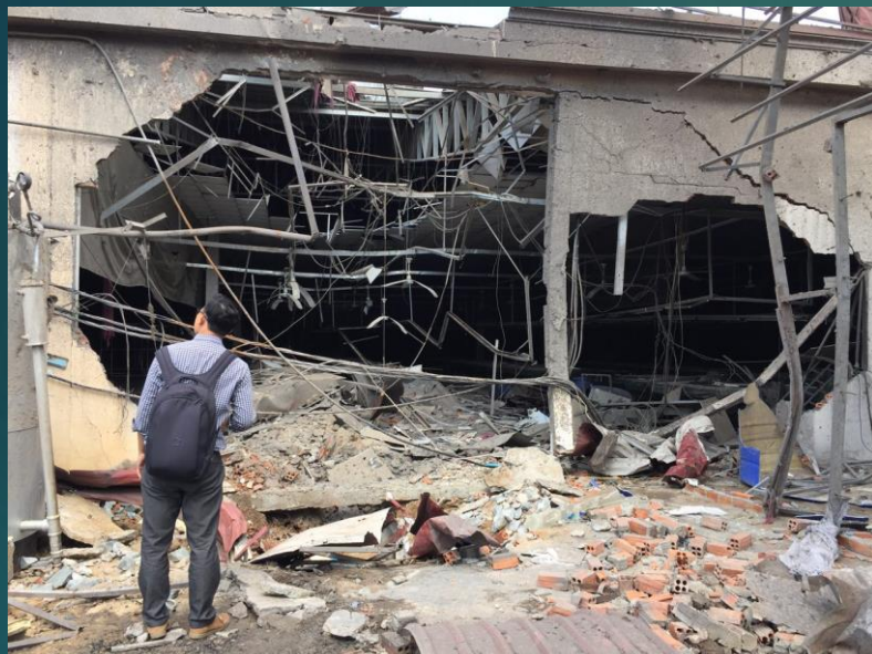
Accident Investigation Boiler explosion
